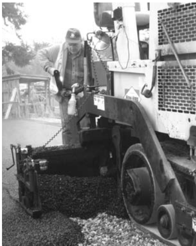
Pervious asphalt, a first for Orcas.
