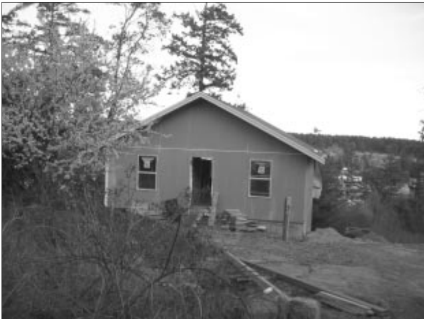
Lahari Ridge home under construction
